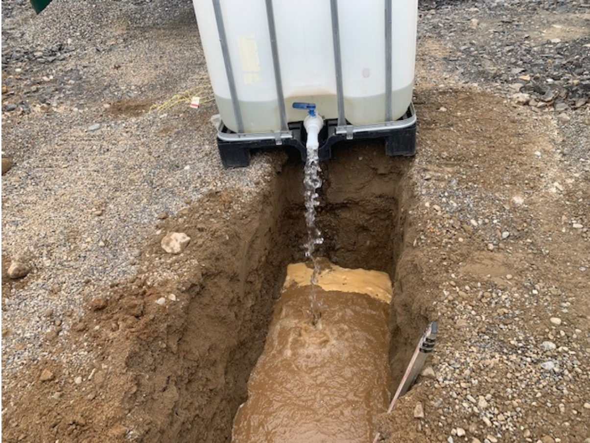
Figure 4:0. Pic showing water discharging quickly into trial pit
